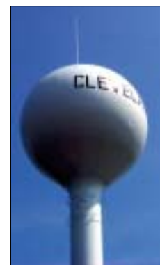
Cell Antenna on Water Tower
