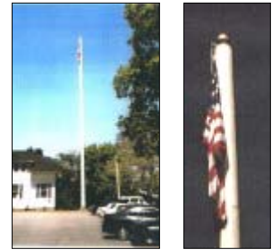
Tower “Flag” Pole Distance & Up- Close Views
